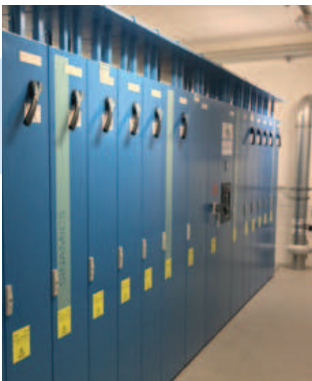
Control cabinets equipped with Sinamics S120 converters and 3WL circuit breakers
