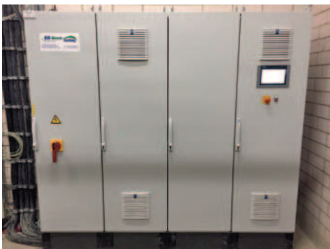
Central measuring, control (MSR) and regulation cabinet based on the Siemens S7 operating instructions
